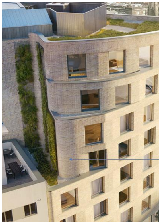
Figure 13: Stainless steel climbers and green roof
